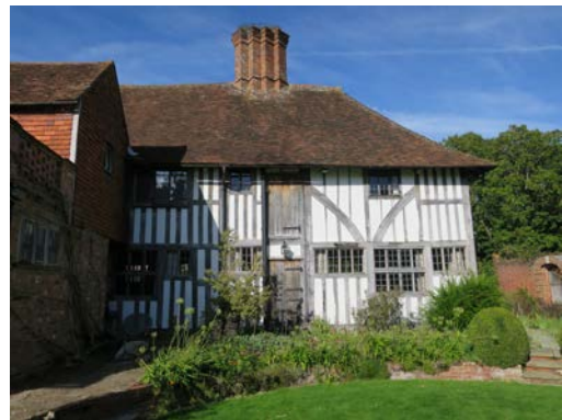
Fig. 2- The rear/ south elevation
