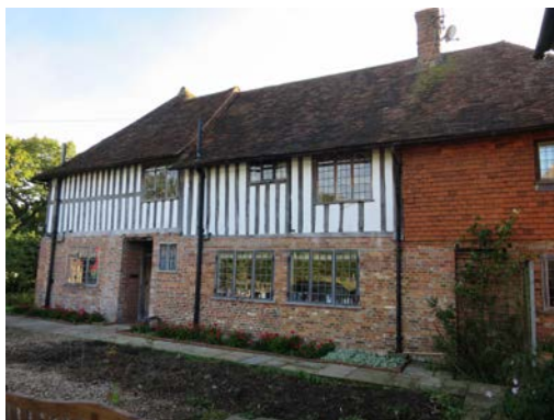
Fig. 3- The west elevation with rear wing
