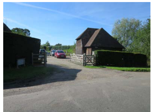
Fig. 4- The driveway and outbuildings
